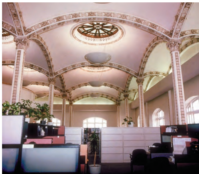
SonaSpray "fc" furnishes this office with a pleasing ceiling finish.
