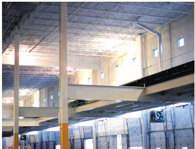
This manufacturing facility utilized K-13 for acoustical control and much needed thermal control.
