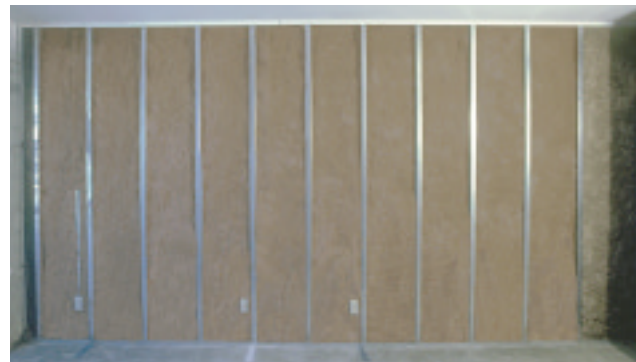
Celbar completely and uniformly fills wall cavities
